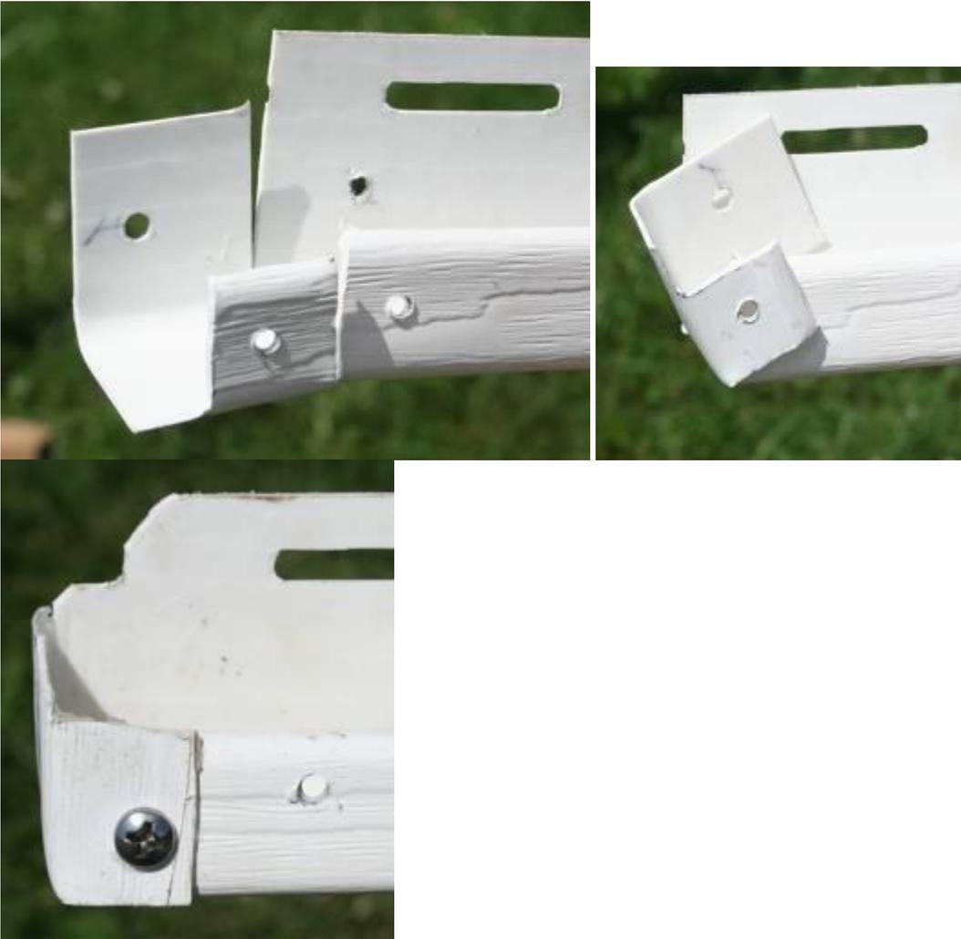
Ends are formed by cutting the "J" channel and bending up to form an end cap. J channel is the material used in vinyl siding on houses.
